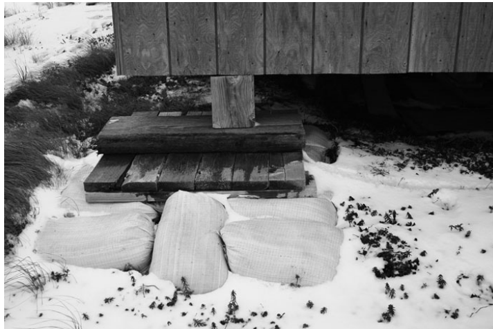
Due to the melting of the permafrost, many homes in Kwigillingok, Alaska, are beginning to sink.
